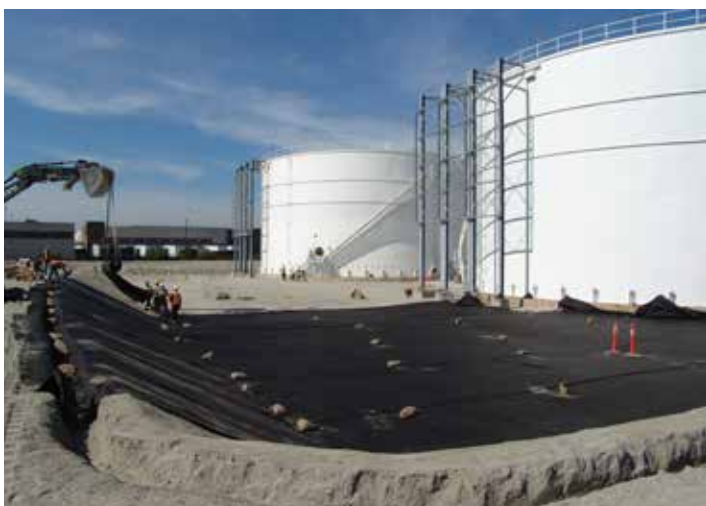
The tanks will have impermeably lined secondary containment areas
